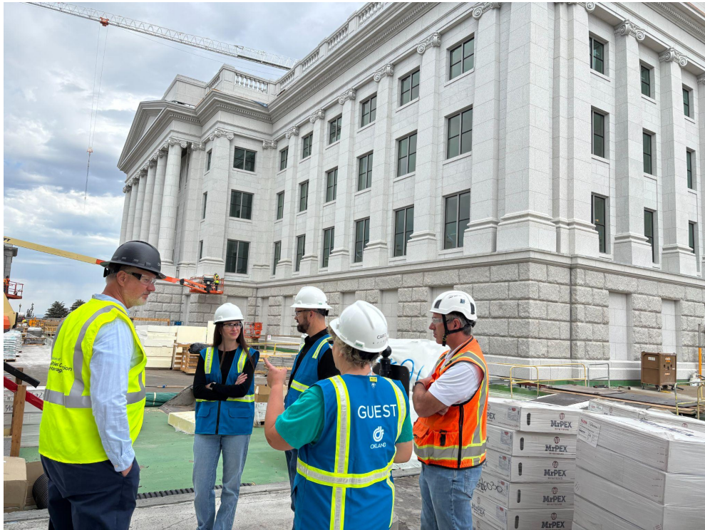
Employees receiving a tour from DFCM and a contractor of the new Michael O. Leavitt Building (North Capitol Building) as construction neared completion.
